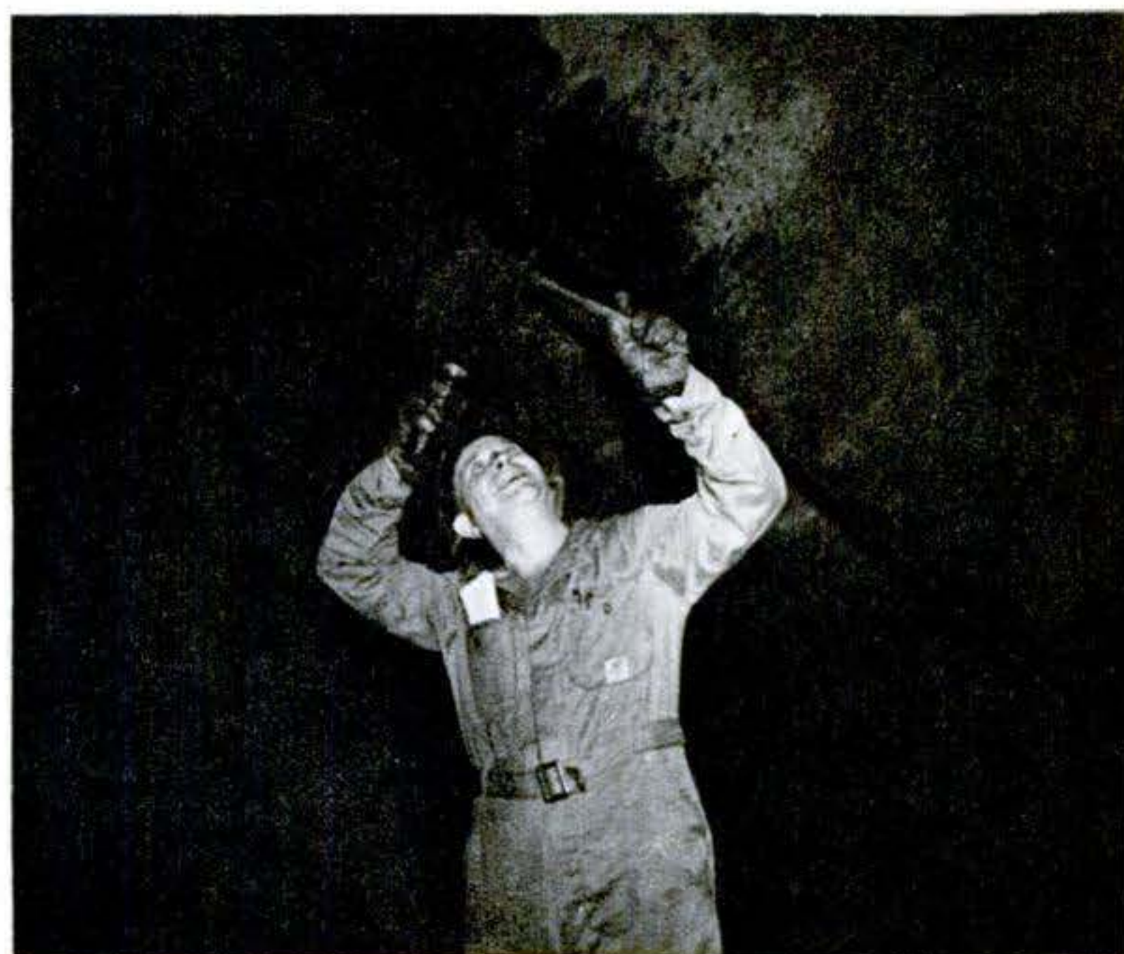
8. Inspector for marine underwriters, with hammer and flashlight, tests welding of bilge keel, or antirolling fin. When hull has passed rigid inspection for seaworthiness, and repainting is done, dry-docking operation is reversed to refloat the ship.
